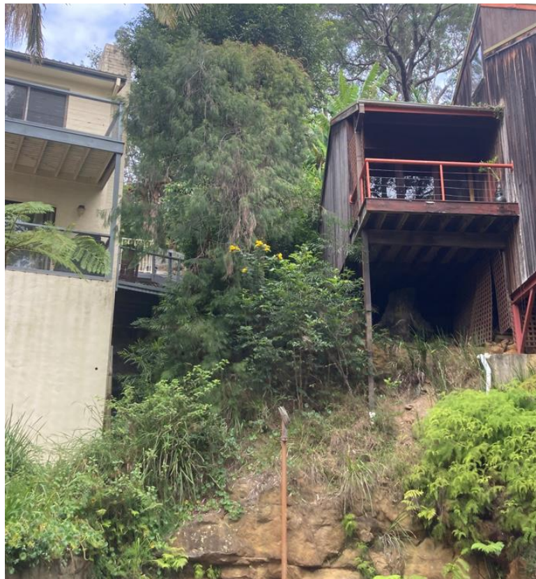
Photo 2: Photo showing natural ground at side
