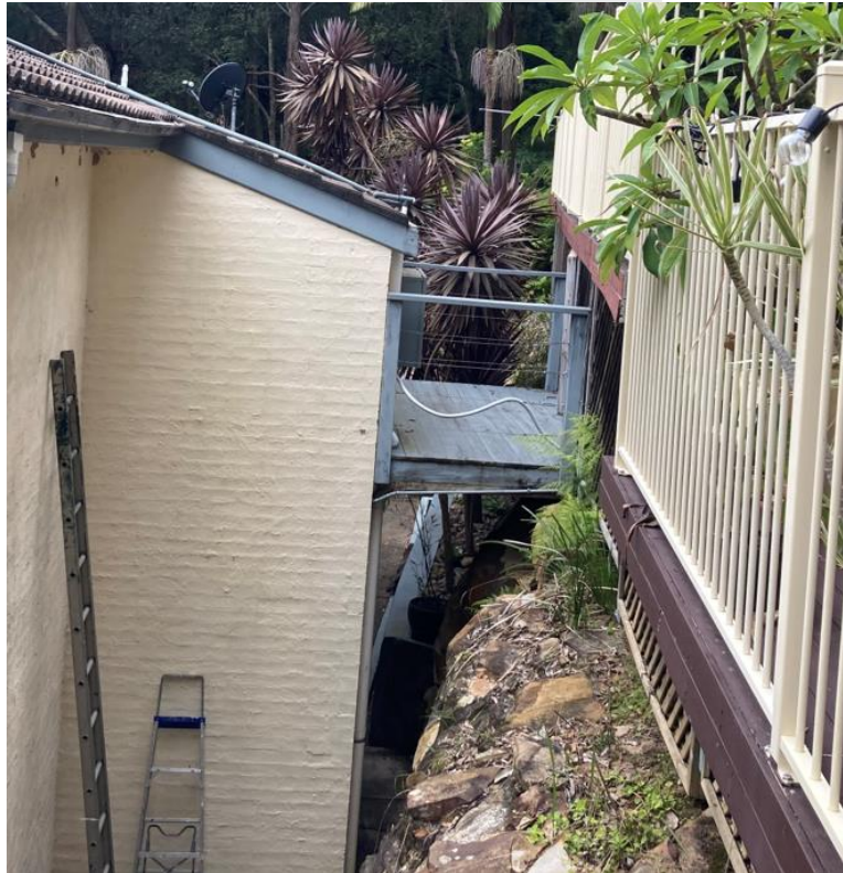
Photo 1: Photo showing natural ground at rear
