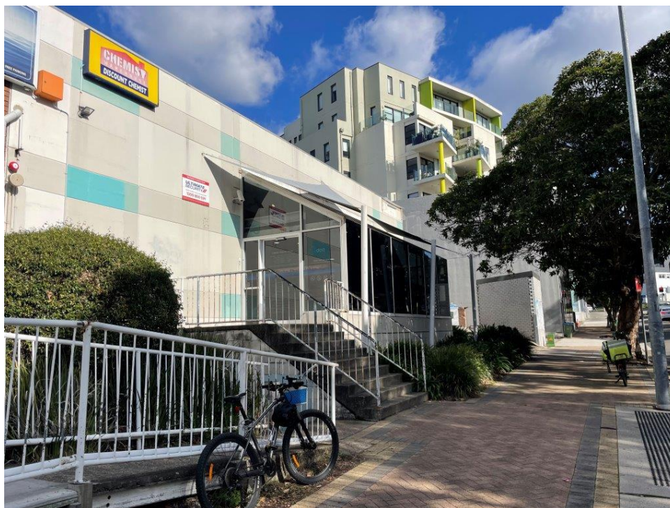
Figure 7 - Dee Why Parade pedestrian entry (ramp and stairs)
