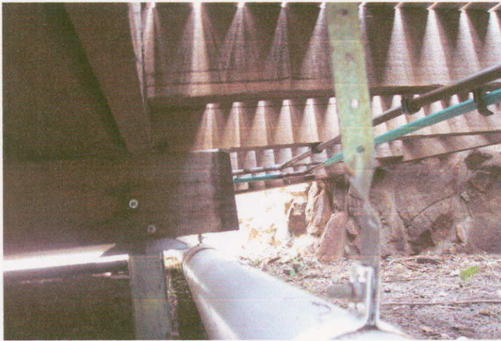
The junction between the extension and the rear deck.
