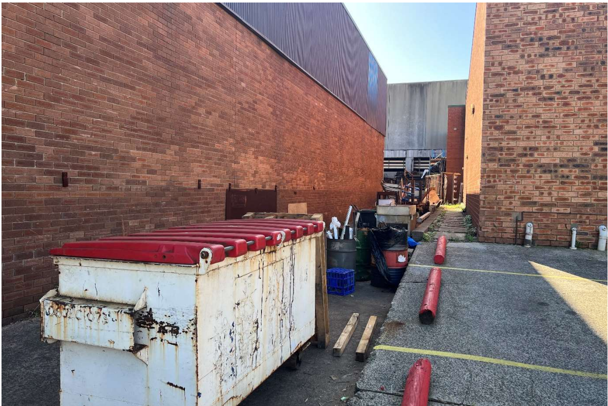
Figure 4 – The eastern side of the building as seen from the front carpark of 12 Boola Place Source: NBP
