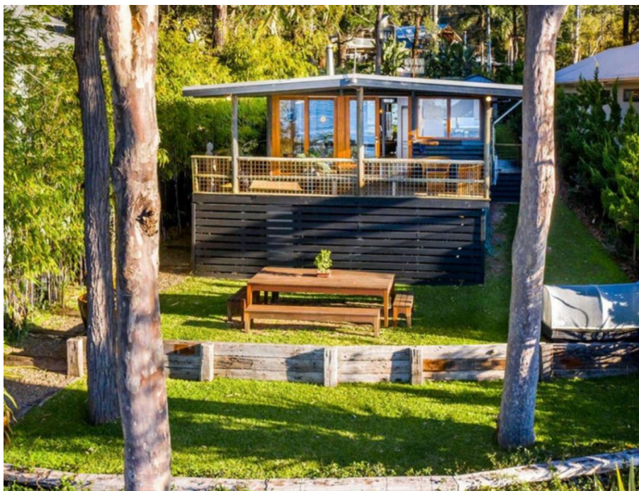
Figure 4. North elevation of dwelling house (source: realestate.com.au)
