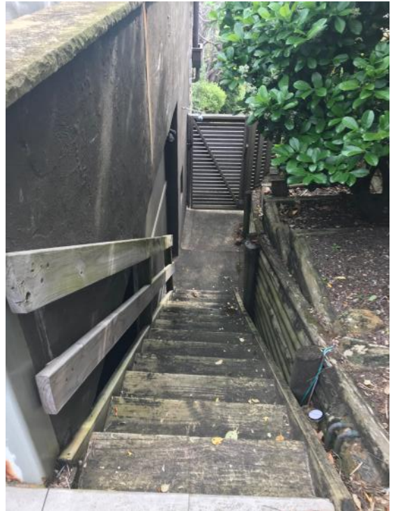
9. Existing stair 03 and retaining wall to northern side passage - to be replaced with metal mesh stair and new retaining walls
