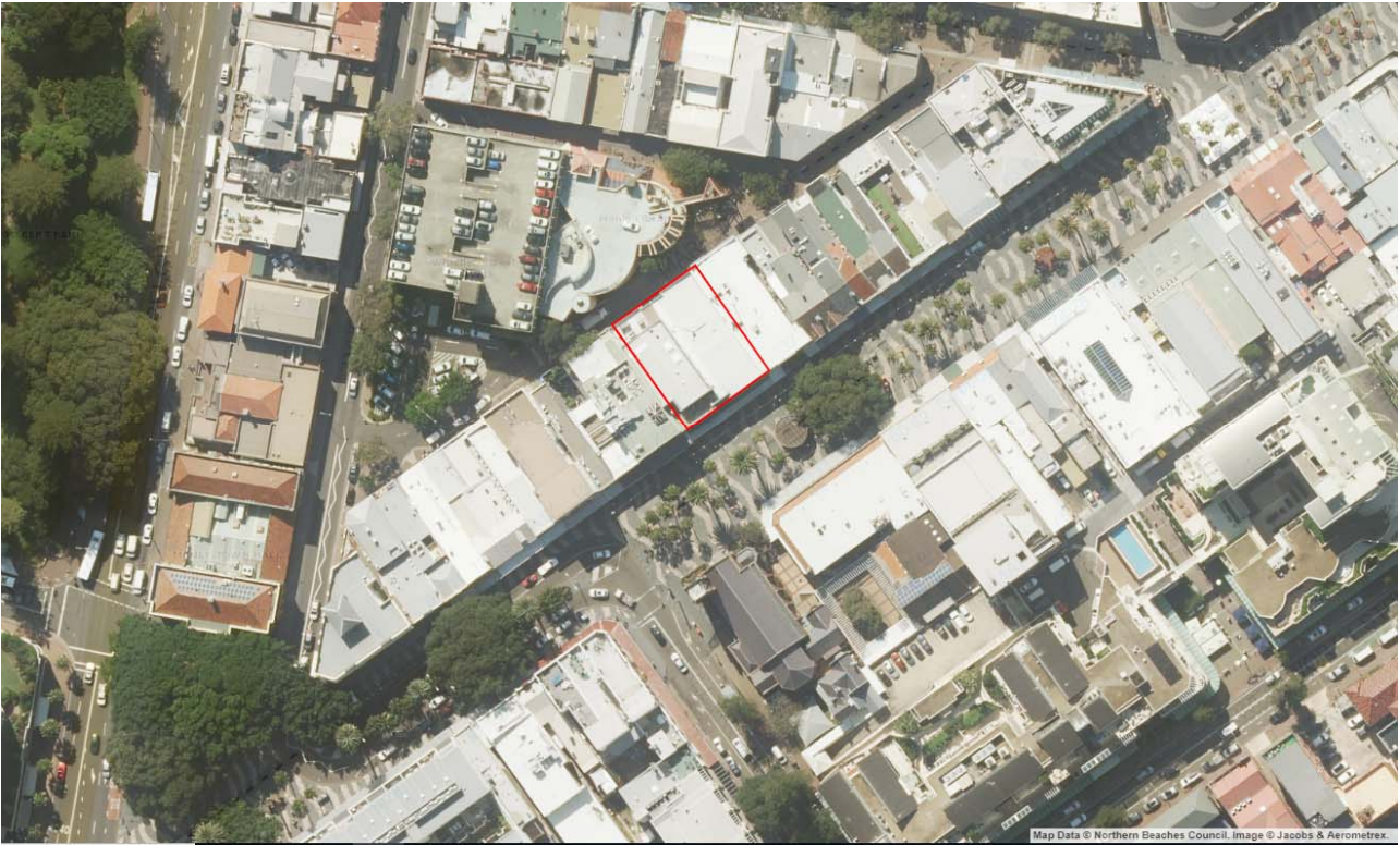
Image – Aerial view of the subject site (courtesy of Northern Beaches Council mapping)
