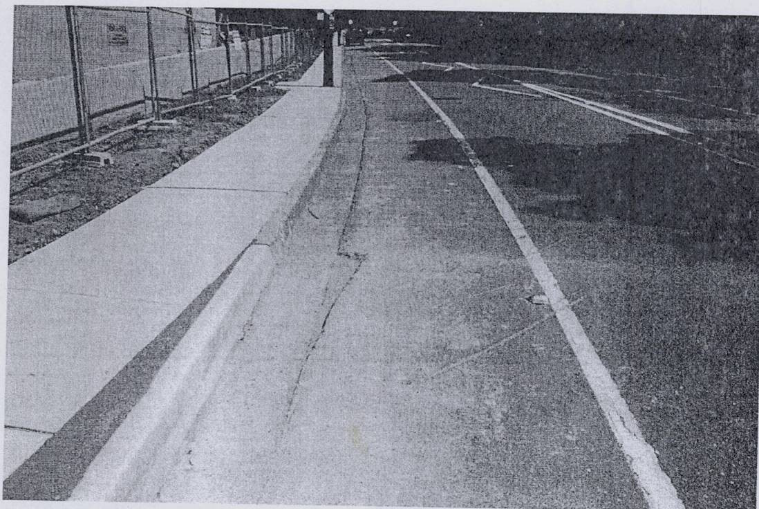
Bayview Golf Club. Adjacent public property. Pittwater Road. Facing north-west along the western side of Pittwater road. Area to the north of power pole no. MV2751. Area compares to photo DSC_0042 & 43 from the original report dated 28.11.07. Section of asphalt missing adjacent to the gutter – area of the previous layback.
