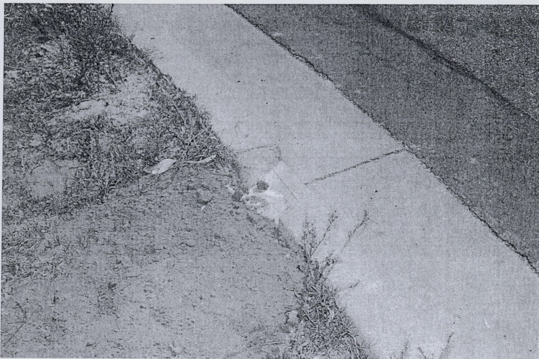
Bayview Golf Club. Adjacent public property. Pittwater Road. Facing north along the western side of Pittwater Road adjacent to power pole no. MV2751. Area compares to photo DSC_0037 from the original report dated 28.11.07. New storm water outlet. Note: no concrete infill above the pipe – check requirements.
