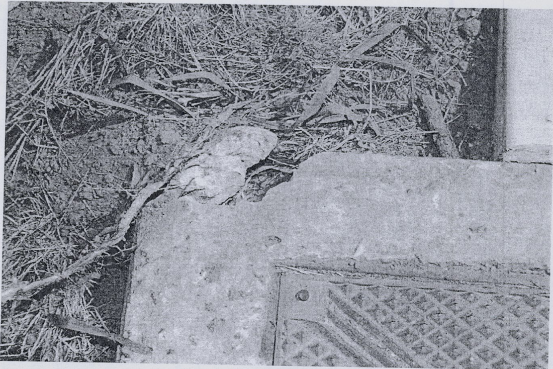
Bayview Golf Club. Adjacent public property. Pittwater Road. Facing north-west along Pittwater Road approaching power pole no. MV2747. Area compares to photo DSC_0051 from the original report dated 28.11.07. Detail of the area seen in the previous photo. Noting the chipped concrete surround to the pit.
