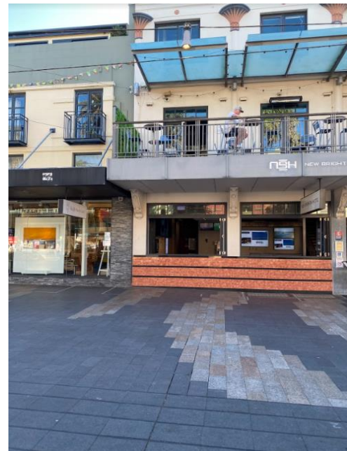
Figure 5 – Interface of NBH and development site Source: Site Inspection, 2022
