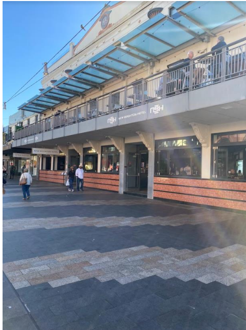
Figure 2 – The New Brighton Hotel (NBH) Source: Site Inspection, 2022
