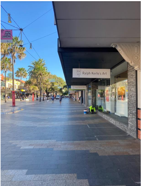
Figure 7 - Awning of development site Source: Site Inspection, 2022
