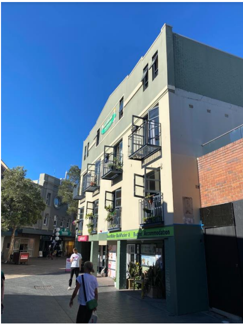
Figure 9 - Rear of development site Source: Site Inspection, 2022
