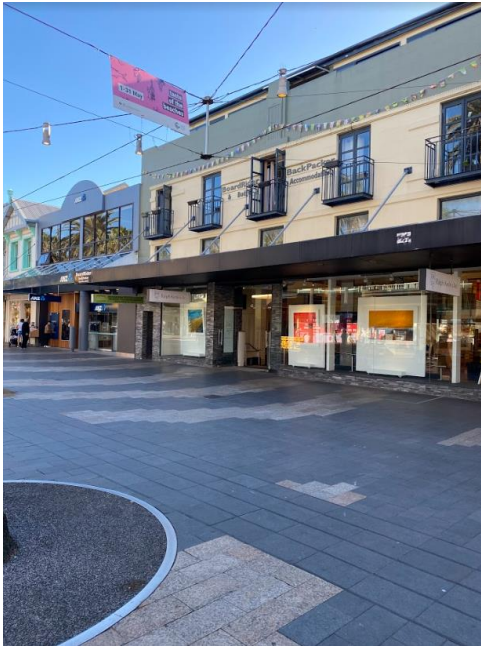
Figure 6 - Development site Source: Site Inspection, 2022
