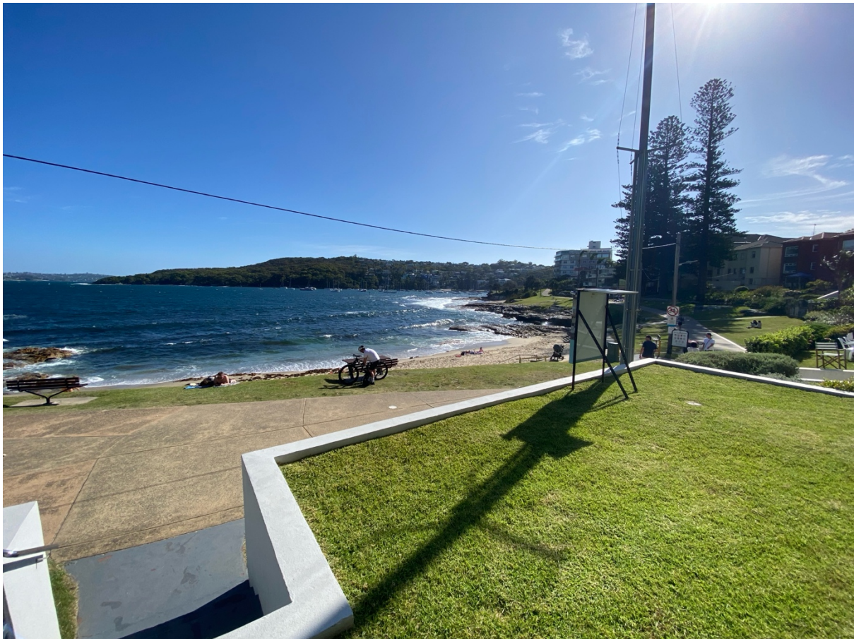
Figure 2: No. 7's Rear Recreation Area (Source: iObject 2024)
