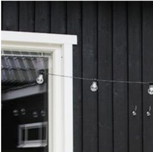
Weatherboard Cladding + Doors/Windows - weatherboard black paint finish - windows/doors white paint finish
