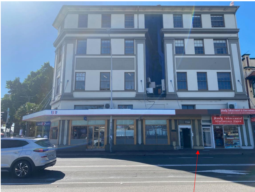
Photograph looking north-east along the East Esplanade frontage – entrance to Lot 20
