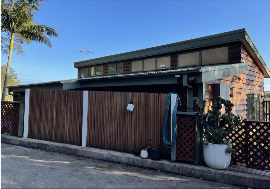
Figure 8: The rear of the existing dwelling, looking south.
