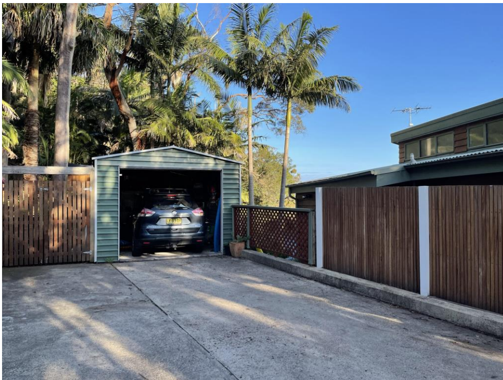
Figure 7: The rear of the existing dwelling and garage, looking east.
