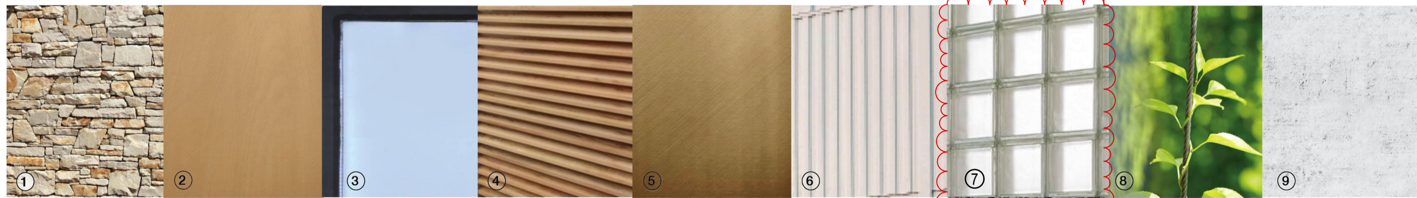
1 Quarried on-site sandstone 2 Render in timber colour 3 Clear glazing & dark metal mullions 4 External venetian louvres 5 Render in bronze colour 6 Light coloured profiled metal 7 Glass blocks 8 Landscaped roof and Ground 9 Smooth concrete
