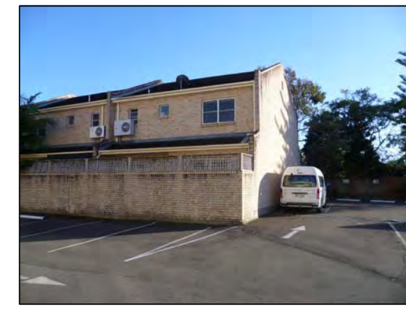
PHOTOGRAPH LOCATION 4 17-19 FORESTVILLE AVE
