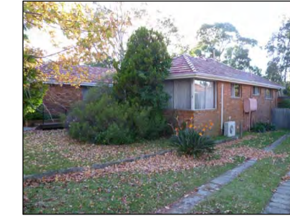
PHOTOGRAPH LOCATION 15 No.35 MELWOOD AVE
