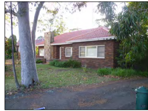
PHOTOGRAPH LOCATION 17 No.37 MELWOOD AVE
