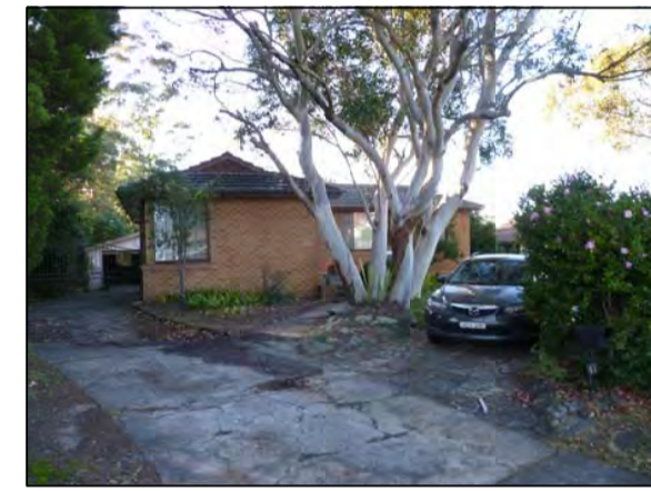
PHOTOGRAPH LOCATION 18 No.41 MELWOOD AVE
