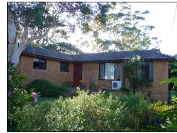
PHOTOGRAPH LOCATION 19 No.41 MELWOOD AVE
