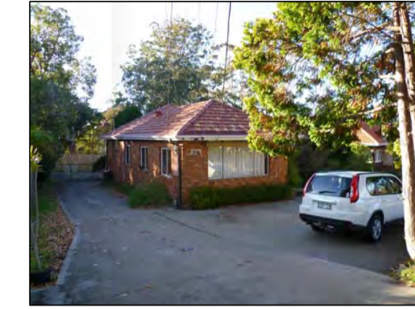
PHOTOGRAPH LOCATION 14 No.35 MELWOOD AVE
