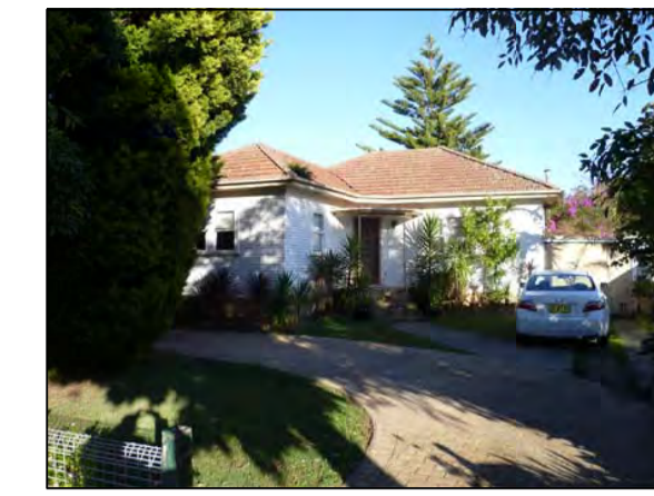
PHOTOGRAPH LOCATION 6 No.18 MELWOOD AVE
