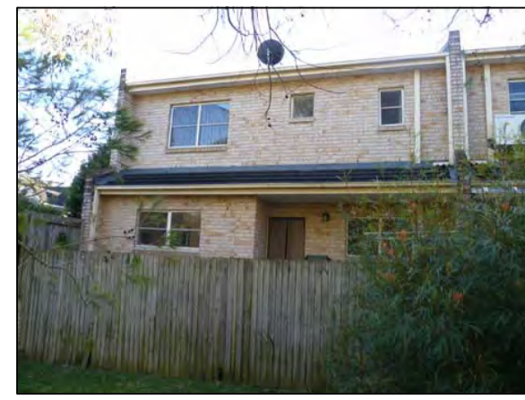
PHOTOGRAPH LOCATION 1 17-19 FORESTVILLE AVE
