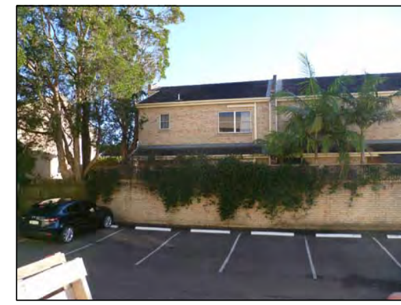
PHOTOGRAPH LOCATION 3 17-19 FORESTVILLE AVE
