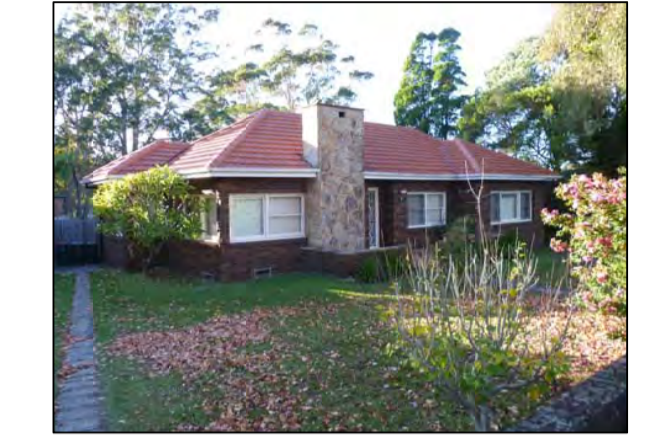
PHOTOGRAPH LOCATION 16 No.37 MELWOOD AVE
