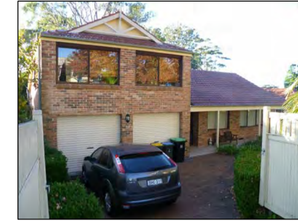
PHOTOGRAPH LOCATION 13 No.33 MELWOOD AVE
