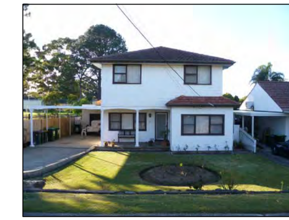
PHOTOGRAPH LOCATION 7 No.23 MELWOOD AVE
