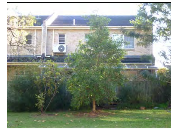
PHOTOGRAPH LOCATION 2 17-19 FORESTVILLE AVE
