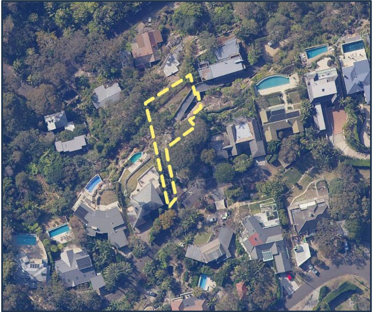
Figure 2: Site Aerial with the subject site outlined in yellow (Source: NSW Planning Portal)
