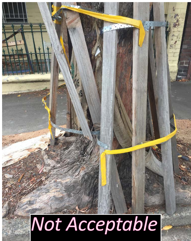
Figure 5. Poor trunk protection.
