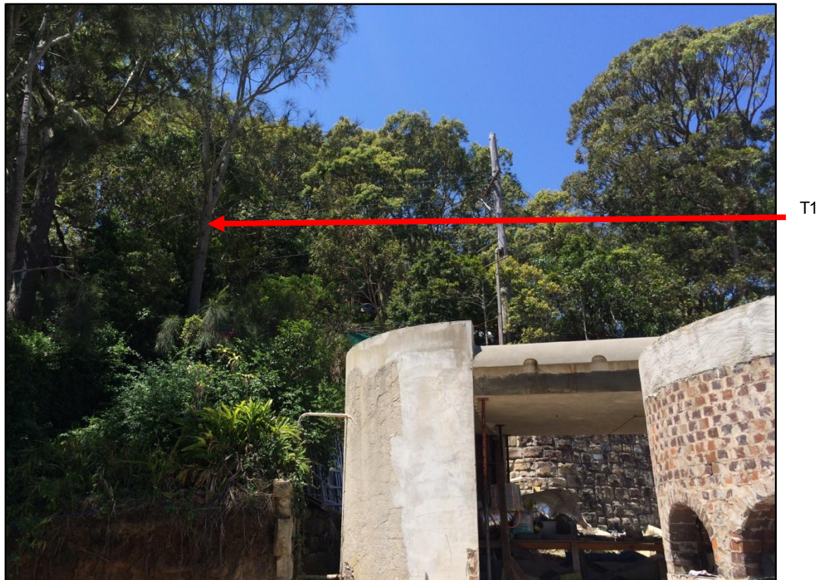
Photo B: Existing features in the vicinity of the proposed Garage (looking northeast).
