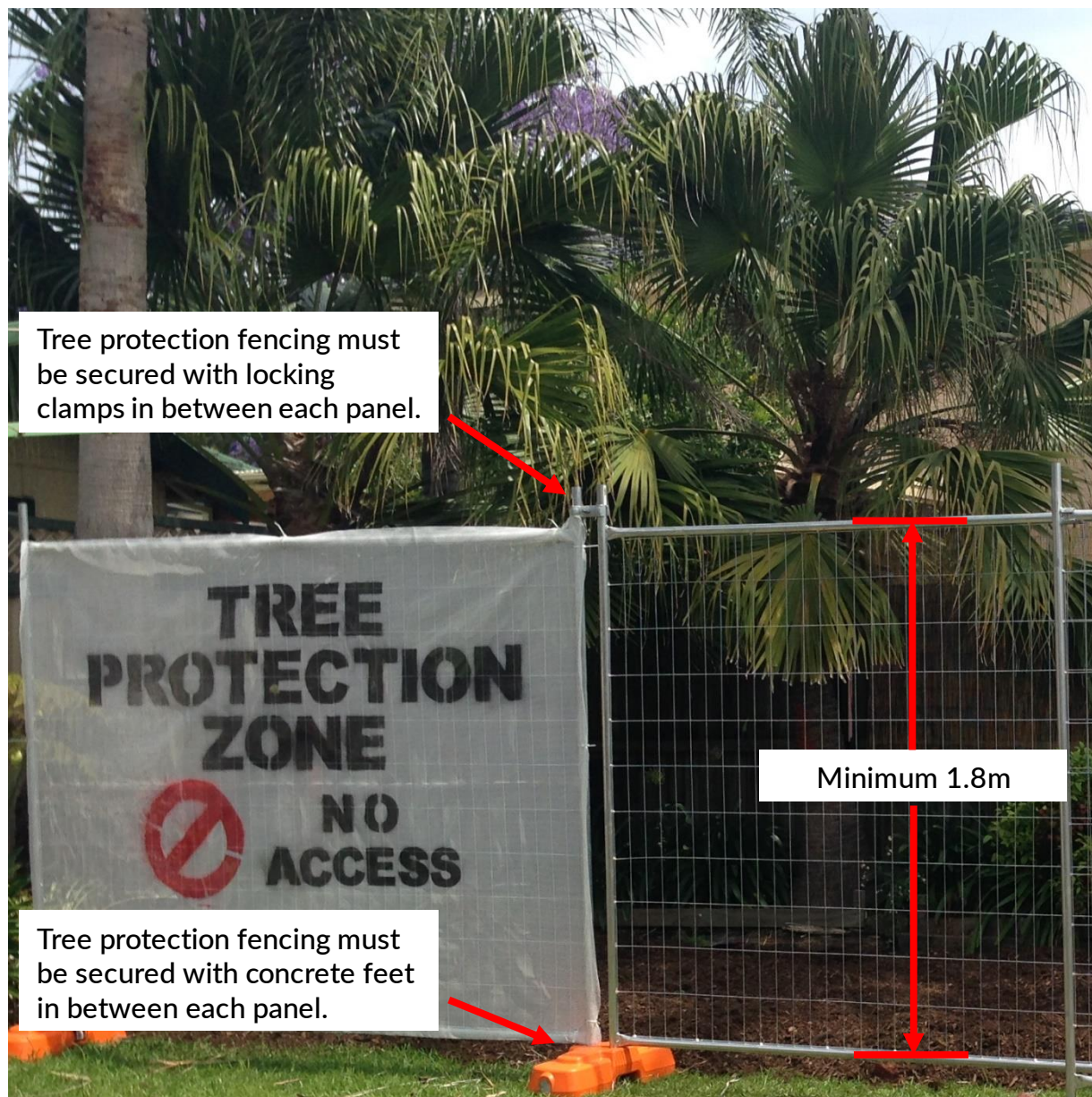
An Example of Temporary Fencing
