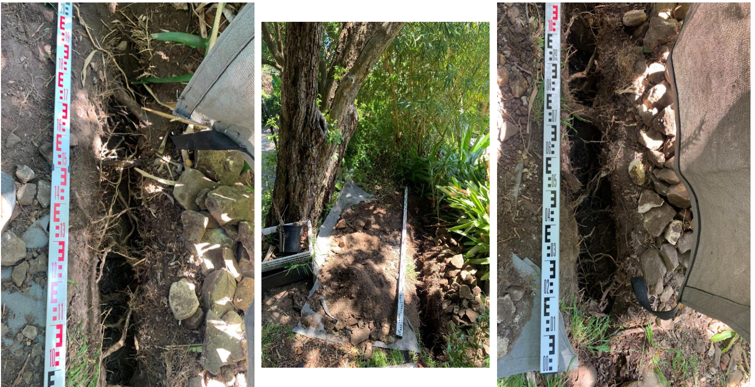
Figure 2: T32 - Preliminary Root Investigation
