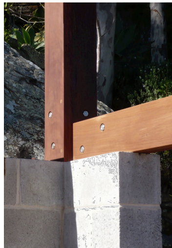
concrete block and hardwood structure to lower ground floor
