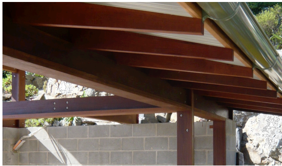
Concrete block and hardwood structure to lower ground floor
