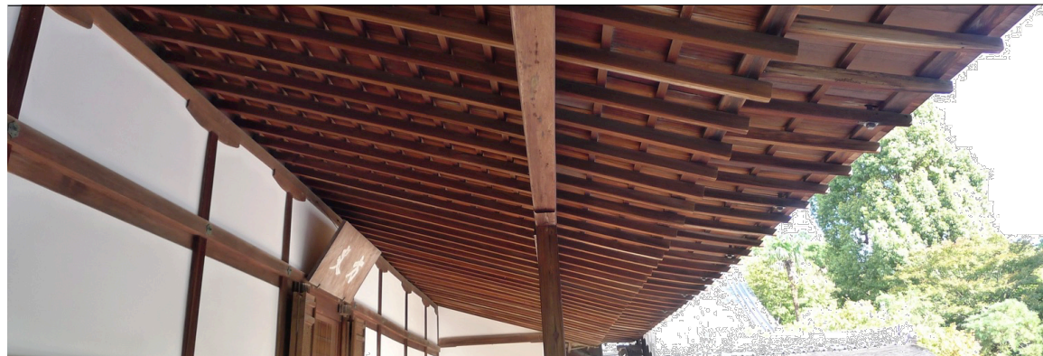
Exposed hardwood roof structure to verandah
