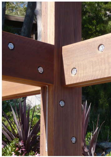
kiln dried tallowood framing with stainless steel bolt fixings
