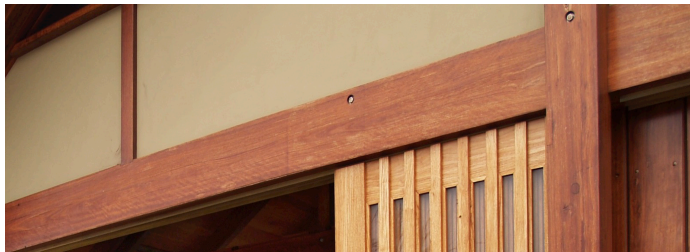
Tallowood hardwood frame, sliding slatted screen, murobond paint on fibrous cement
