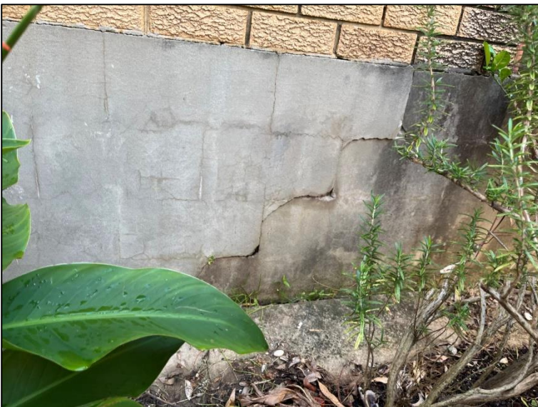
Photograph 6 – Step cracking
