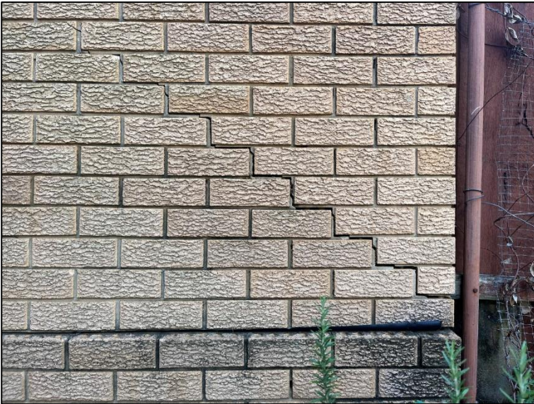
Photograph 5 – Step cracking
