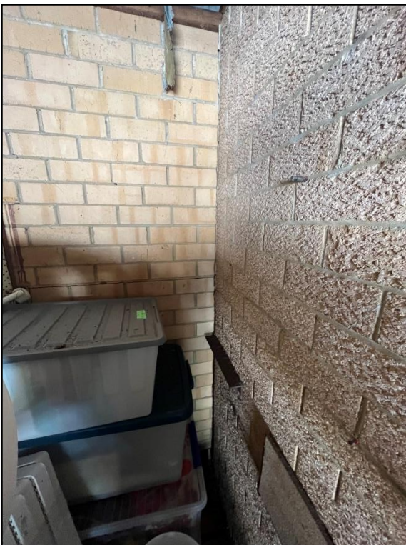
Photograph 2 – Overview of rear garage wall and partition wall
