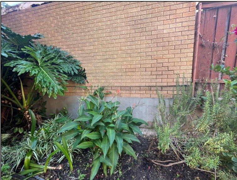
Photograph 4 – Overview of retaining wall
