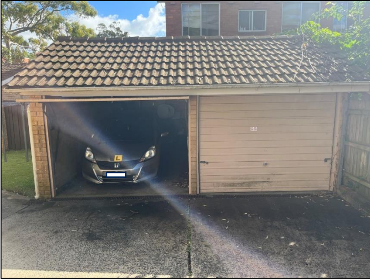
Photograph 1 – Overview of two-tenancy garage
