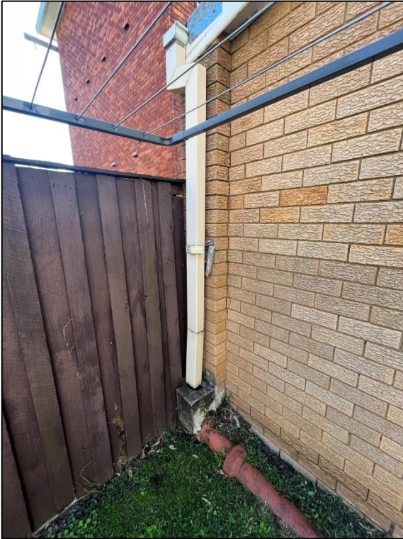
Photograph 9 – Overview of clay pipe and water system
