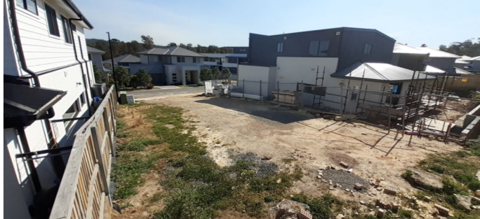
IMAGE 01 - SITE IMAGE OF THE REAR OF THE BLOCK
