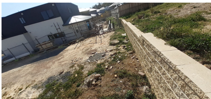
IMAGE 03 - SITE IMAGE OF THE REAR RETAINING WALL
