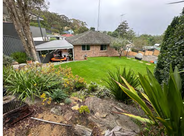
Photo 2: Rear of the dwelling facing north-east.
