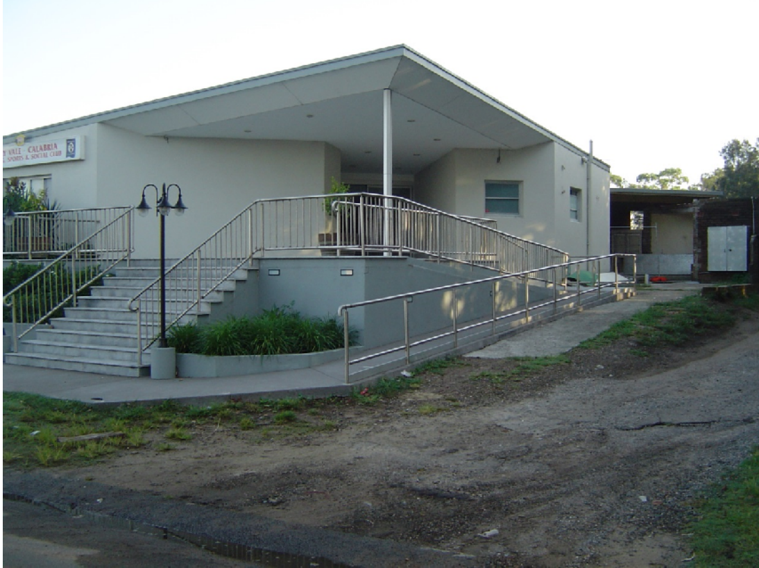
Front elevation that shows the main entrance and ramp that is as built
