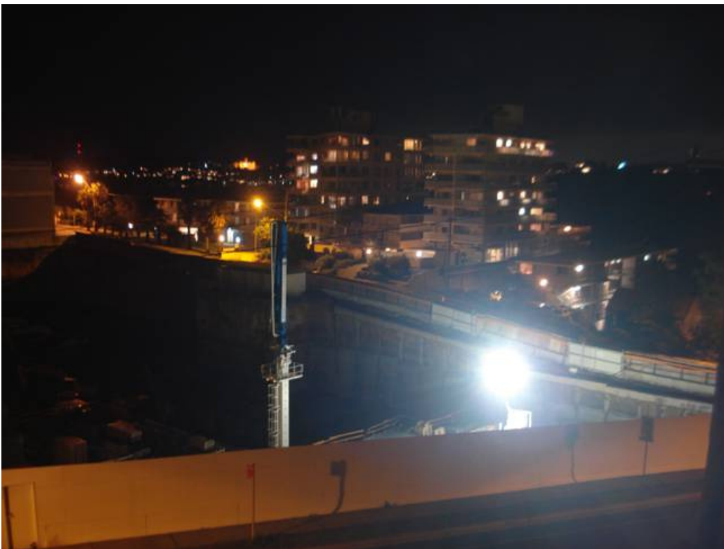
Photo of work at HDC on 23/11/2016
