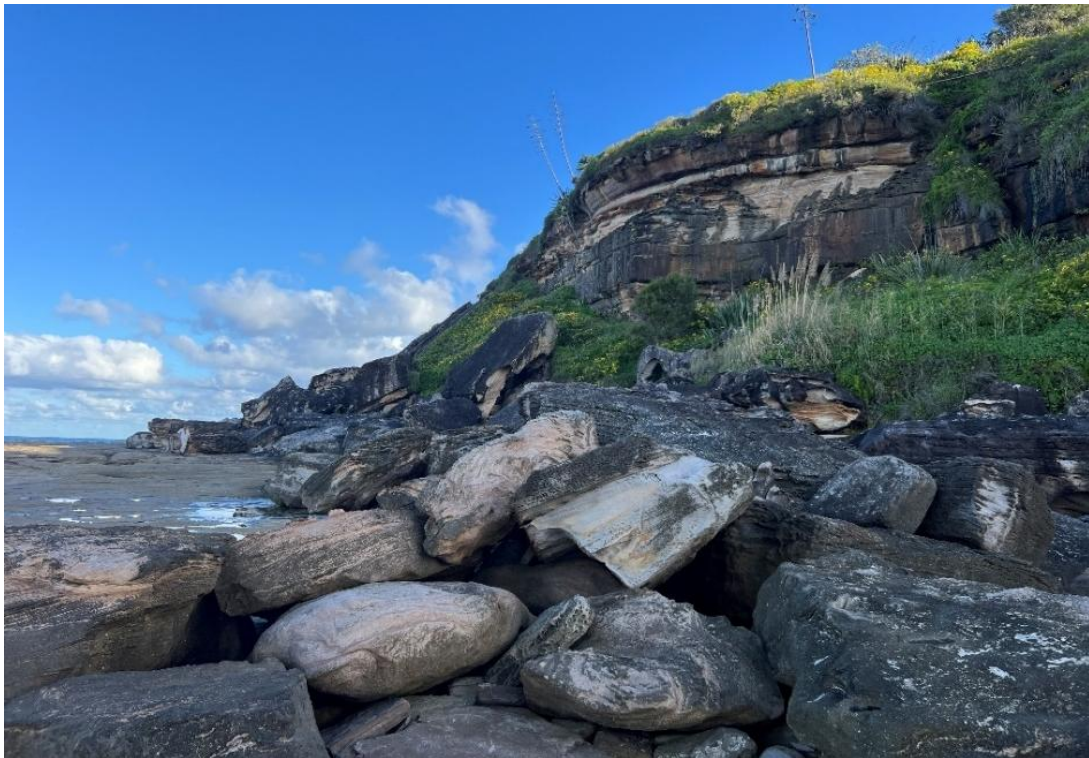
Figure 4-3 Boulder armour at the cliff toe
