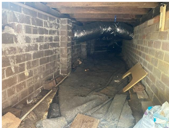
Photograph: 5 – showing subfloor brick footing walls.
