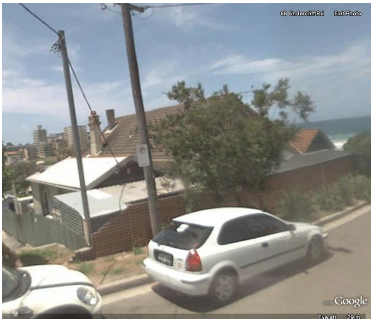
Photograph 1: Pilu Restuaurant as viewed from Undercliff Street.
