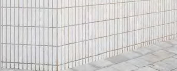
vitrified white wall tile (ie 80x240) to inside and outside face of rc up-stand element of balustrade on upper deck - and the proposed stack bond look in context
