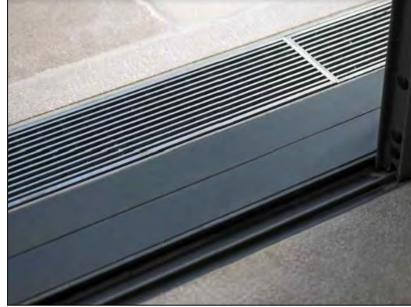
example of stainless steel slot drain to front of stacking sliders b/w new enlcosed room and open balcony
