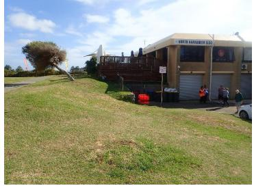
Figure 14. Western side of SLSC building showing cut into the adjoining land (looking north)
