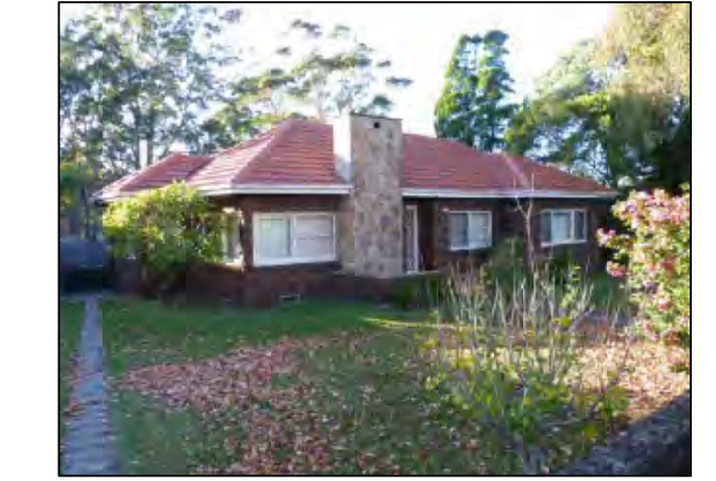
PHOTOGRAPH LOCATION 16 No.37 MELWOOD AVE
