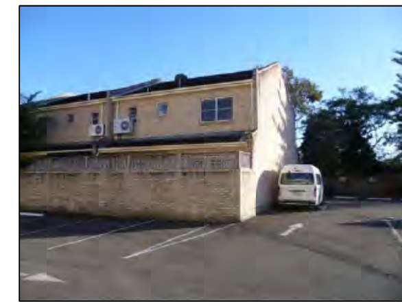
PHOTOGRAPH LOCATION 4 17-19 FORESTVILLE AVE
