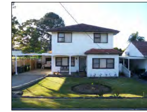
PHOTOGRAPH LOCATION 7 No.23 MELWOOD AVE
