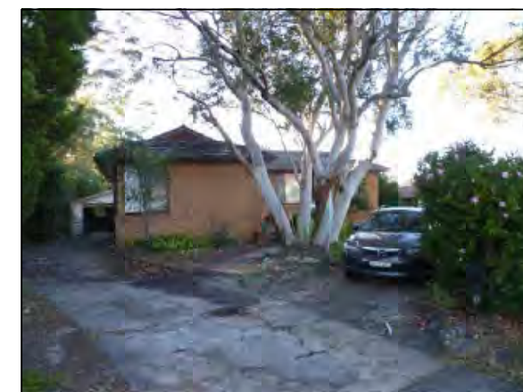
PHOTOGRAPH LOCATION 18 No.41 MELWOOD AVE
