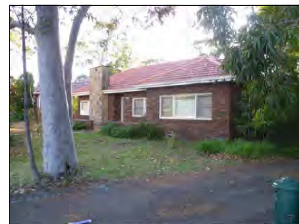
PHOTOGRAPH LOCATION 17 No.37 MELWOOD AVE
