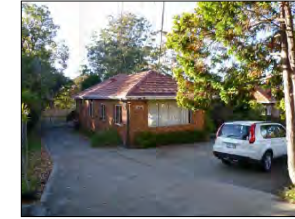
PHOTOGRAPH LOCATION 14 No.35 MELWOOD AVE
