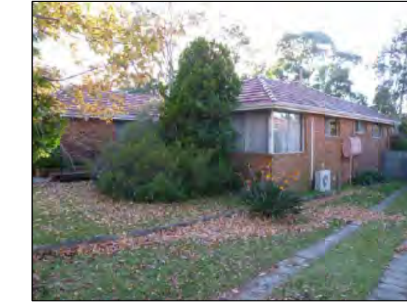
PHOTOGRAPH LOCATION 15 No.35 MELWOOD AVE
