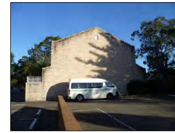
PHOTOGRAPH LOCATION 5 17-19 FORESTVILLE AVE
