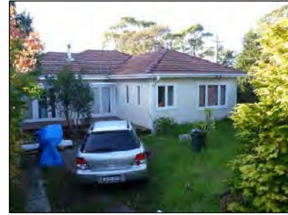
PHOTOGRAPH LOCATION 9 No.27 MELWOOD AVE
