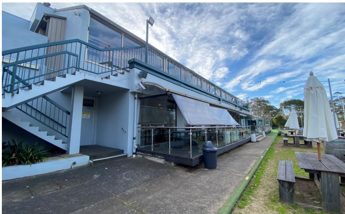
Plate 3 – View towards the north-east showing the back of the RSL Club.
