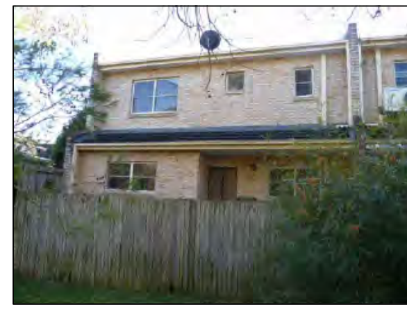
PHOTOGRAPH LOCATION 1 17-19 FORESTVILLE AVE
