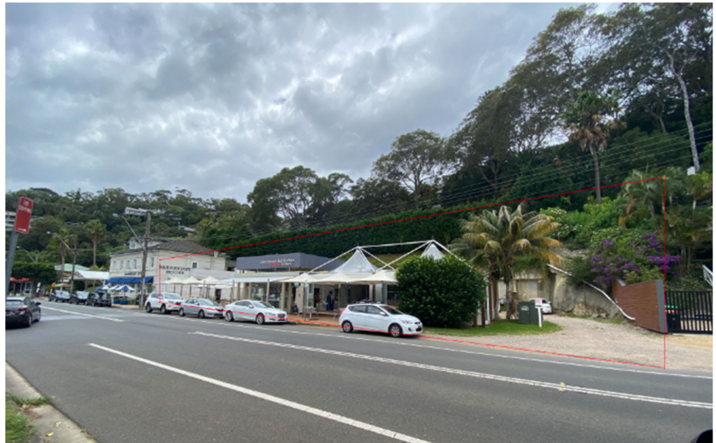
Image 4- View of subject site from south of Barrenjoey Road
