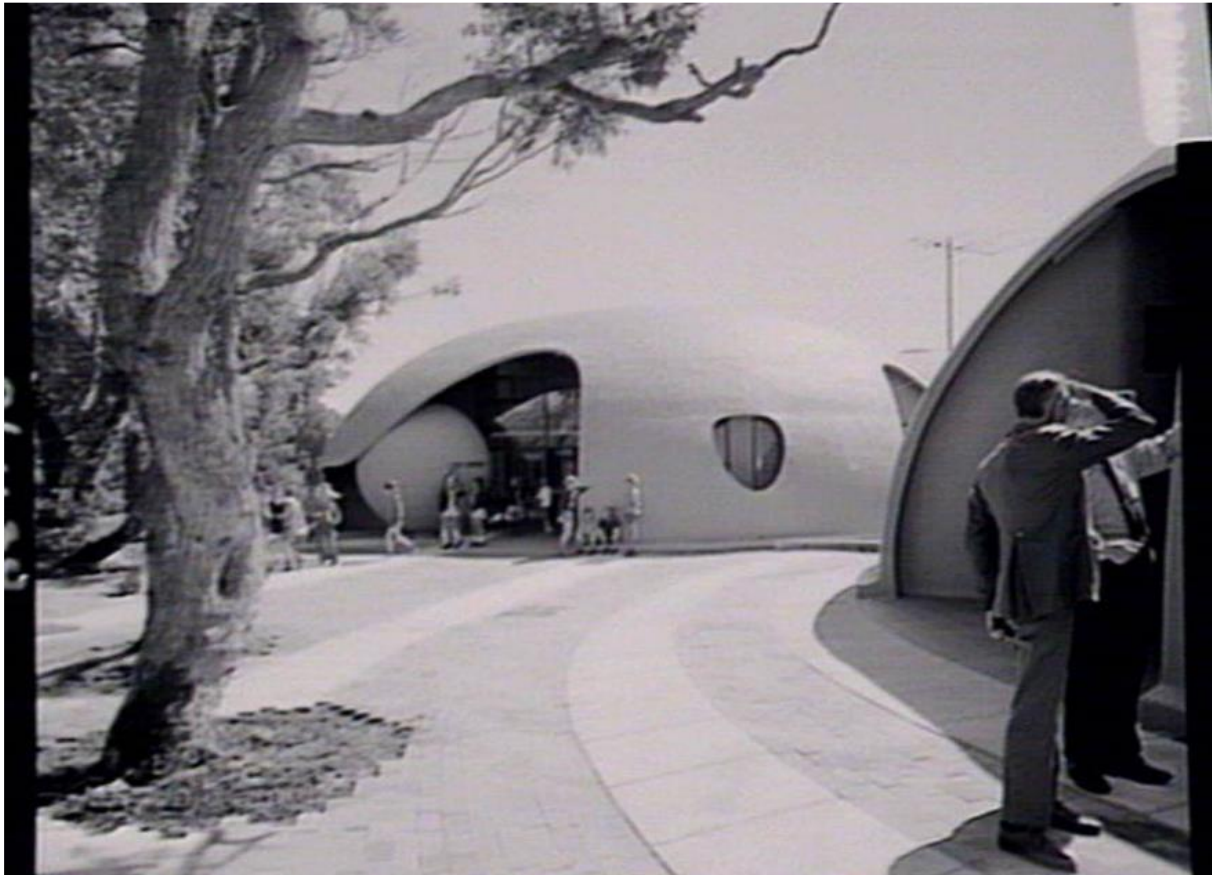
Figure 47: North Narrabeen Public School Binishells, 1975 (Source: NSW State Archives and records, GPO 2 - 47287, File No. FL2347486).
