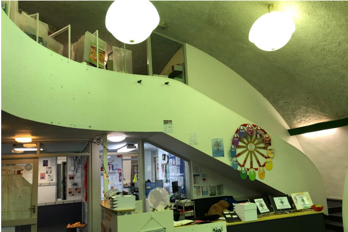
Figure 20: Front dome with administration at ground floor and storage at the upper floor level.
