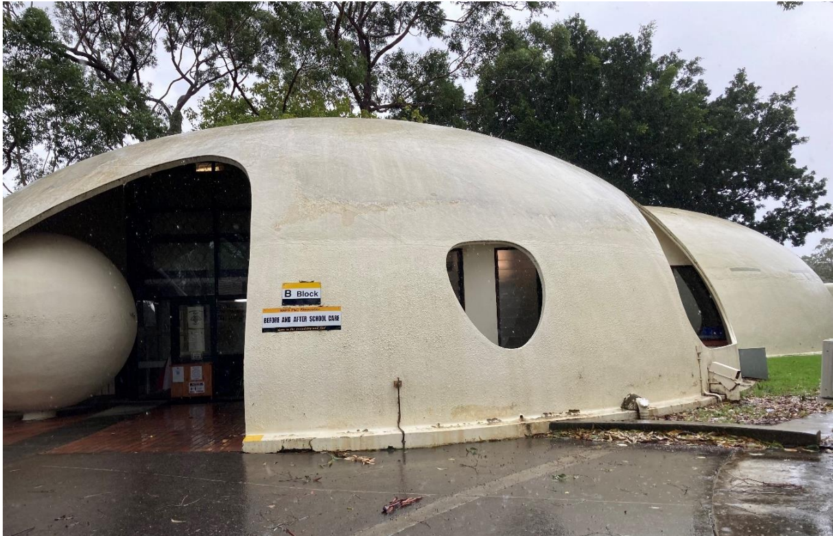
Figure 12: Primary entrance of Bini Shell B, view looking northwest.
