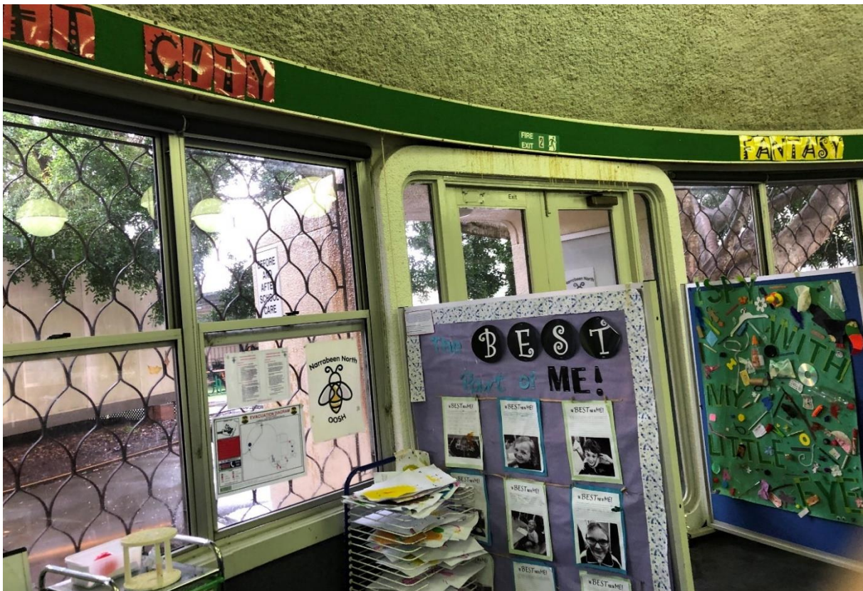
Figure 24: Existing secondary door and window openings at Bini Shell B, view looking northwest.
