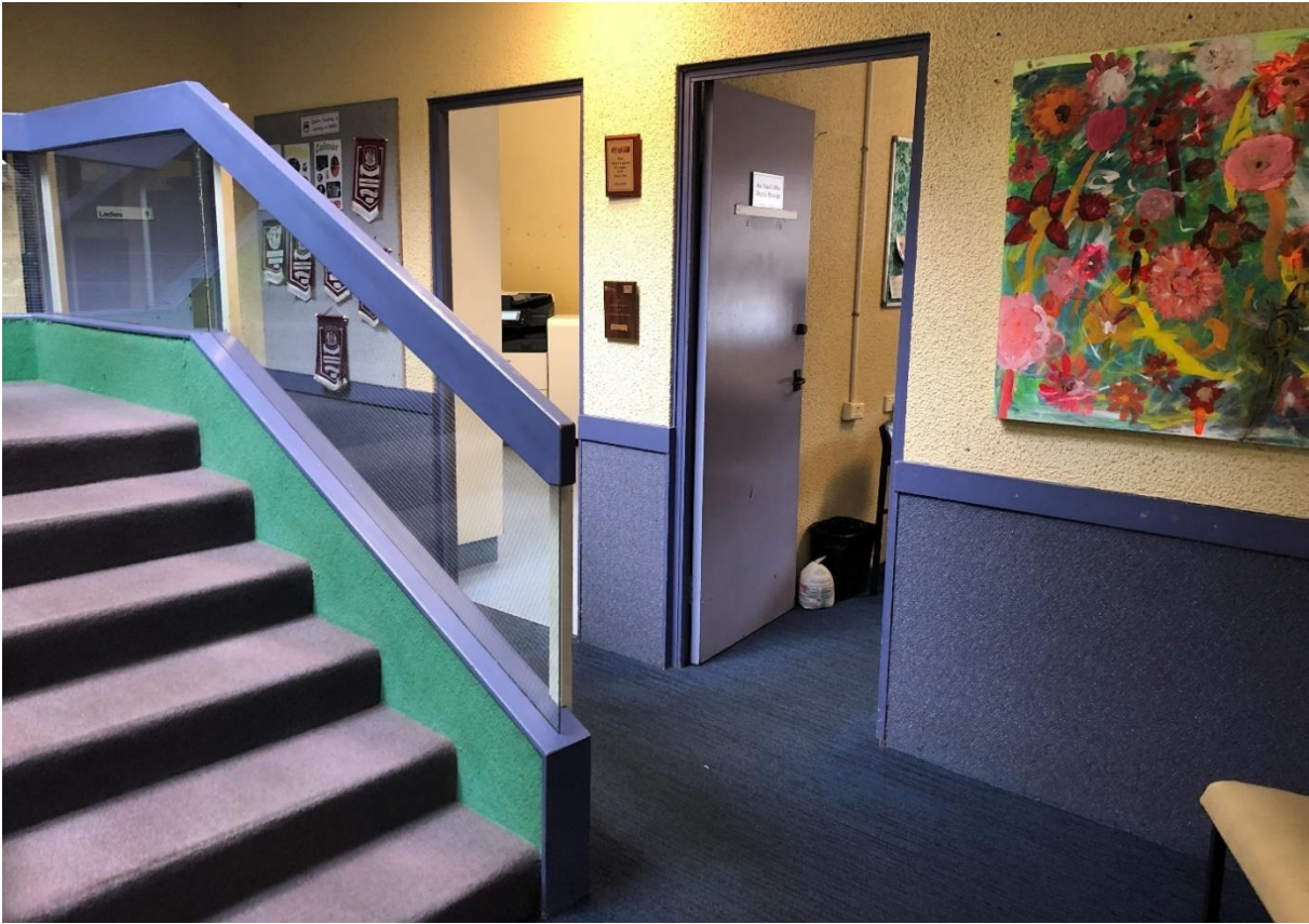
Figure 16: Staircase at Bini Shell A located adjacent to the enclosed courtyard space.
