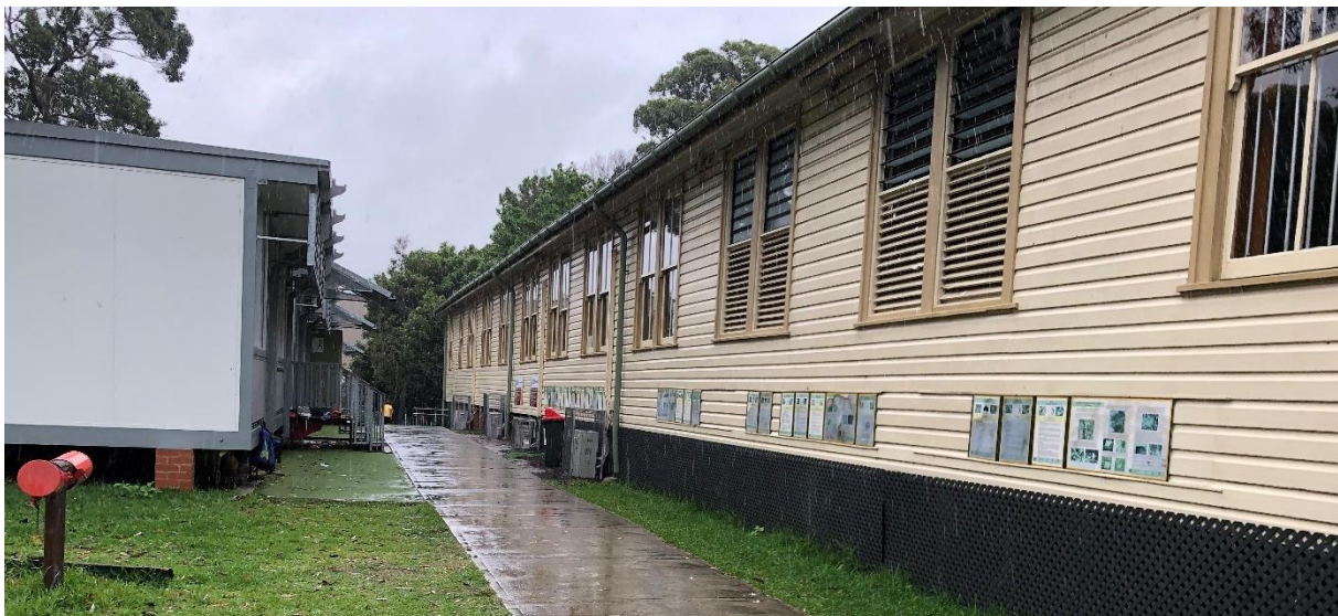
Figure 4: View of Building J and Demountable located south of the Narrabeen North Public School, view looking northwest.
