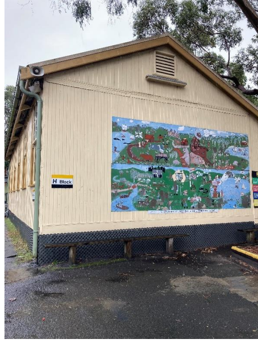
Figure 8: View of Building H (weatherboard), view looking west.
