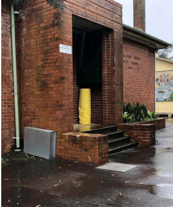
Figure 7: View of Building K (facebrick), view looking southwest.
