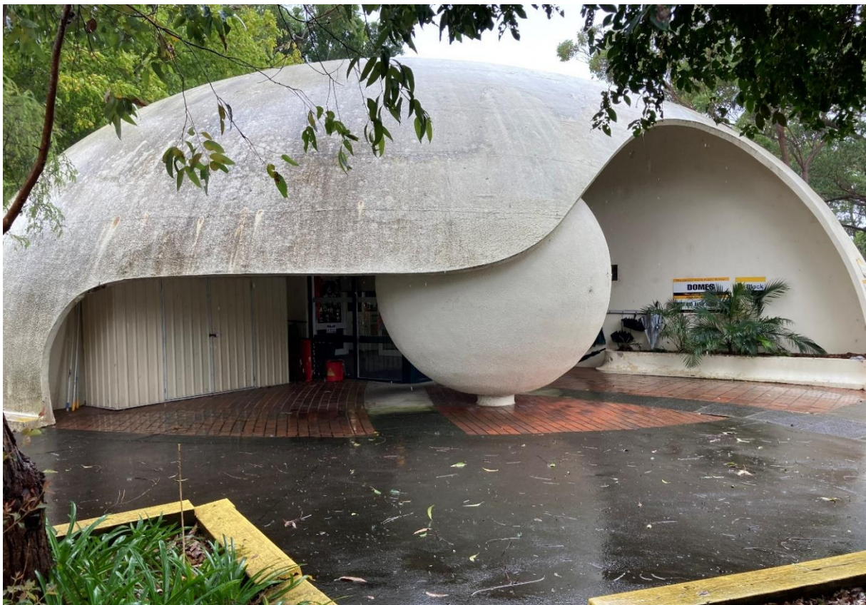
Figure 13: Primary entrance of Bini Shell B, view looking northeast.
