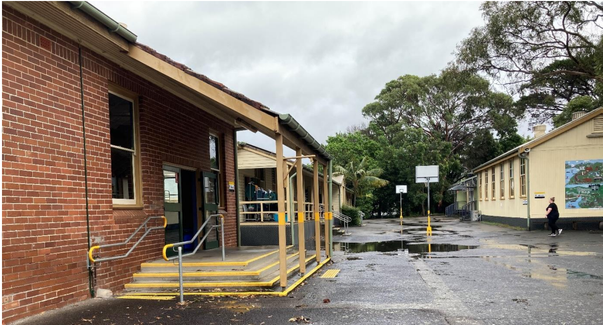
Figure 5: View of Building K (left) and Building H (right), view looking west.
