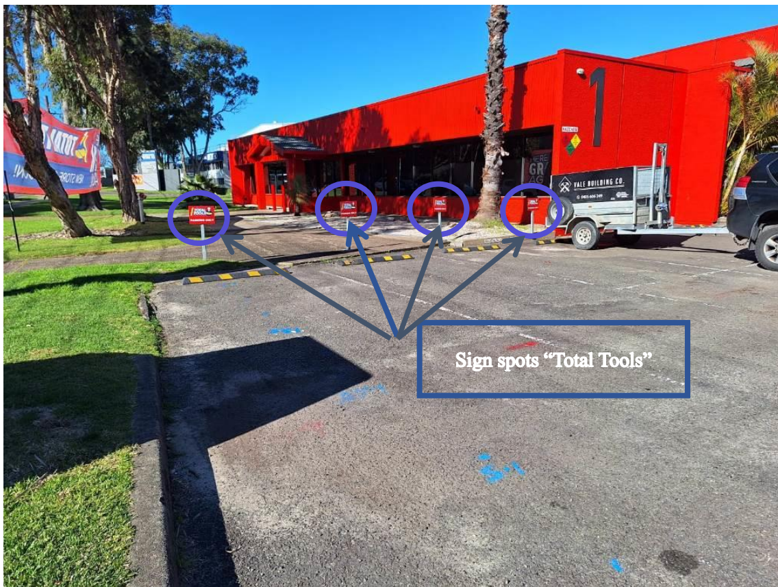
Building as is, including signed car parking "Total Tools". DA not approve yet.
