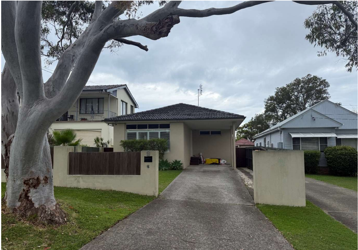
Figure 3 – The subject site (centre) as seen from Blandford Street Source: NBP
