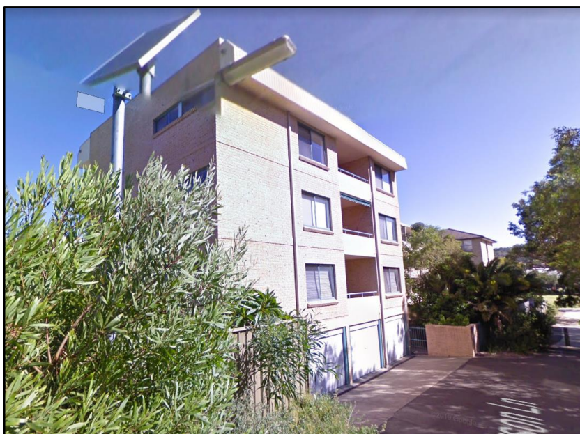
Figure 3 – Rear of apartment building at 65 Old Barrenjoey Rd.
