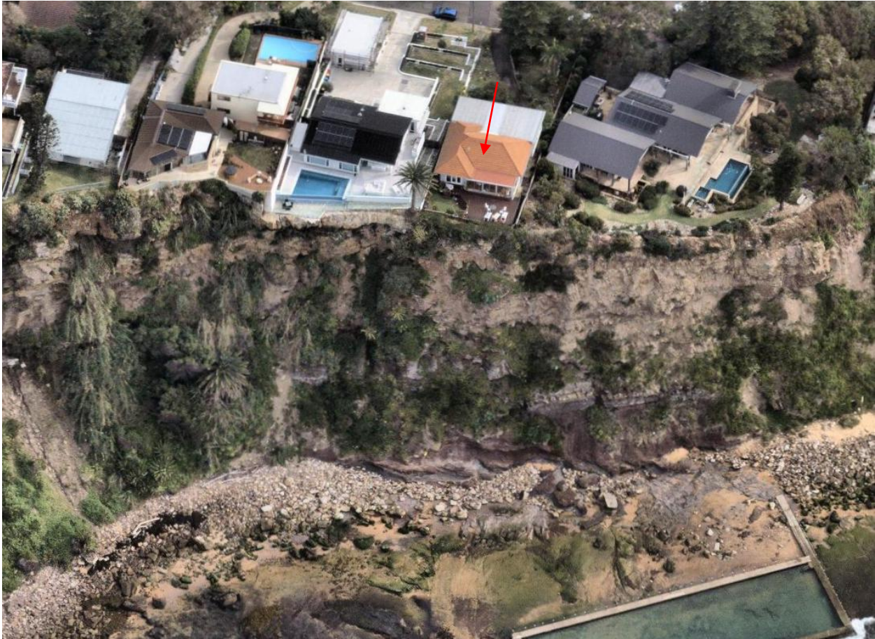
Figure 2: Oblique aerial view of site (at arrow) on 22 July 2024, facing west
