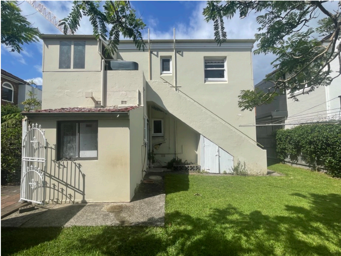
The rear facade of No.67 Eurobin Street showing the single storey laundry under the skillion roof and the second (rear) stair to the first floor unit.
