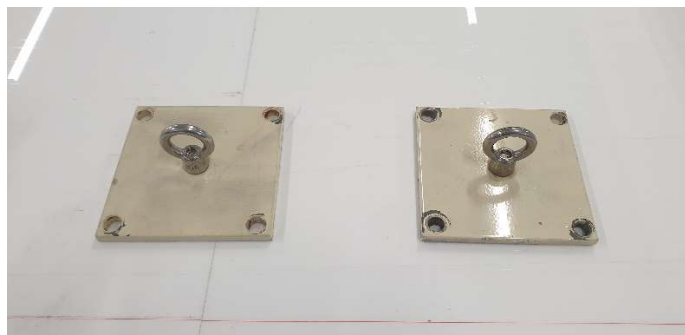
Figure 10 - Typical anchor point plates. The plates will be painted to match the painted and rendered brick wall behind so as to diminish any visual impacts. (Source: Client)
