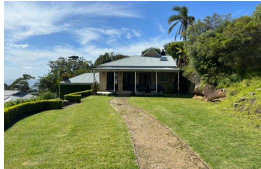
Photo 2: Front of existing dwelling, single storey sandstone block cottage with attached awning. Sandstone outcropping on the southern side of the dwelling, looking east.
