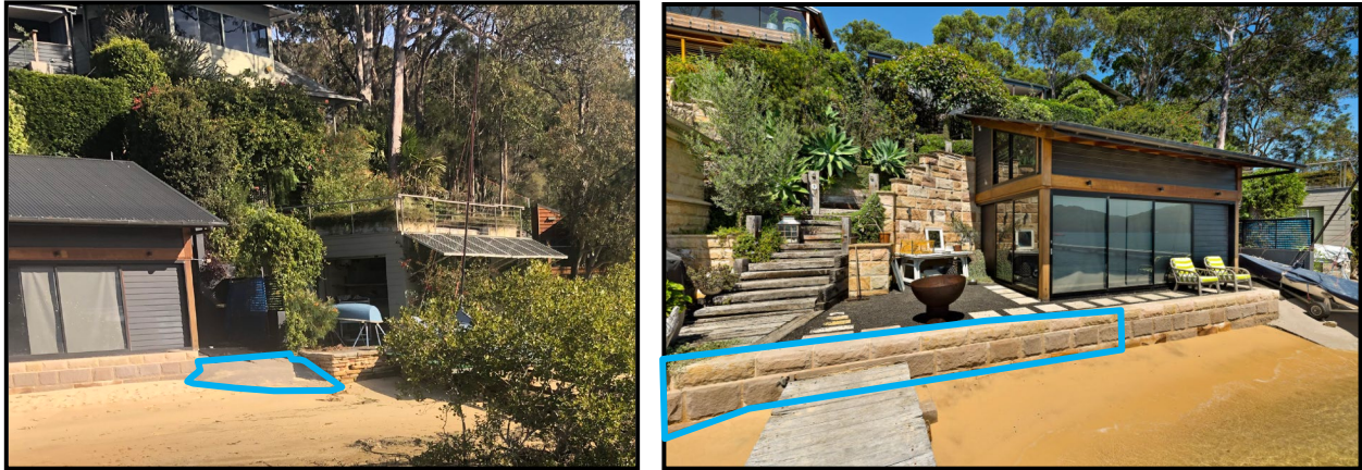
FIGURE 7 Photo depicting the concrete ramp (R) and the sandstone seawall with reclamation (L) subject to the current BICA
