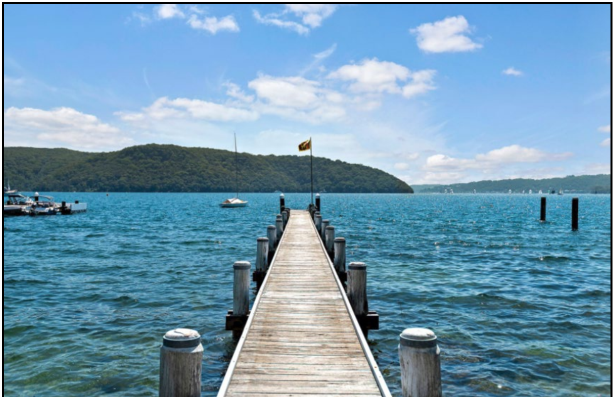
Seaward view of existing water recreation structure, taken from the end of the jetty.
