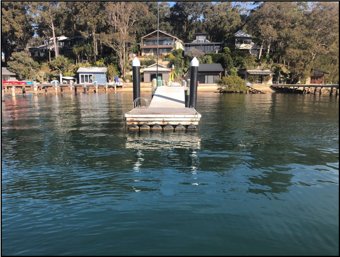
Landward view of existing water recreation structure with residence situated in the background.
