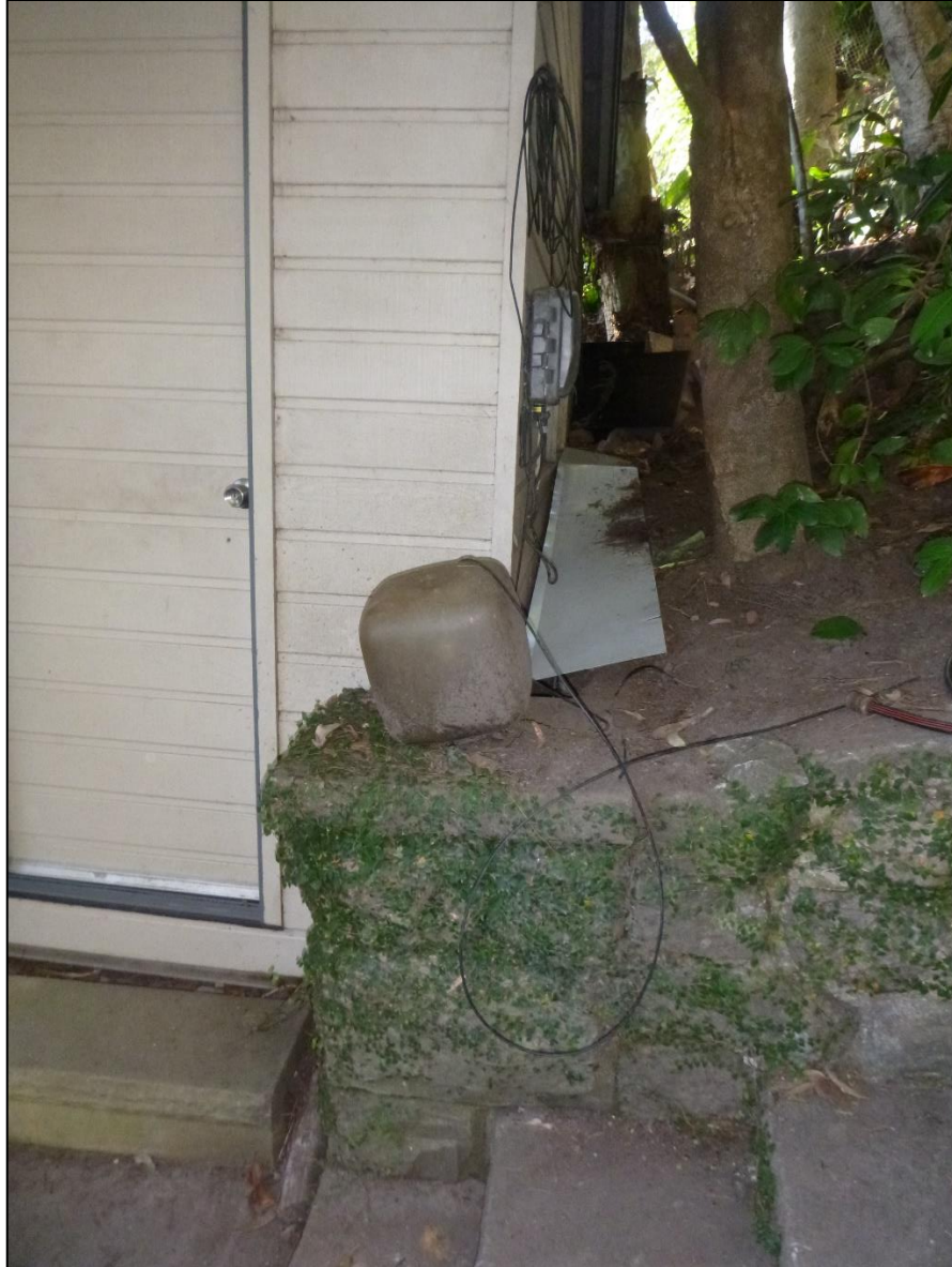
Photo A: Existing retaining wall downslope of Trees 104, 105, 107
