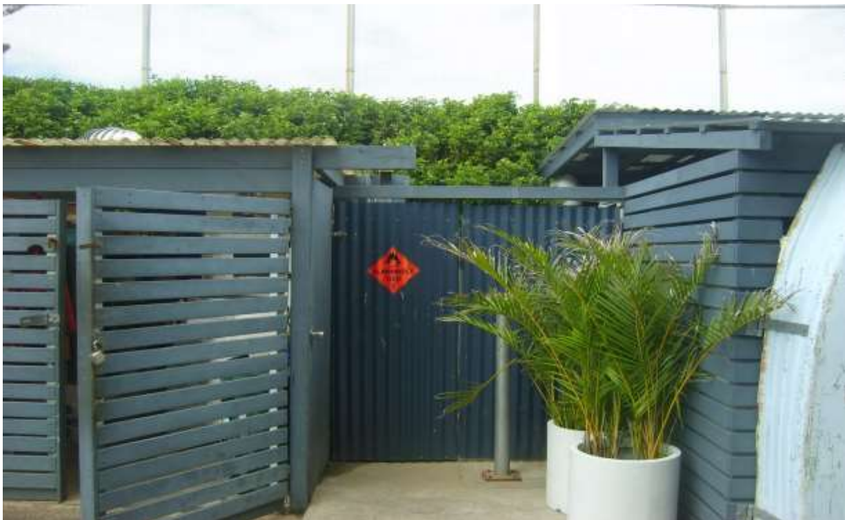
Photo 7 – Indicates the storage facility for LPG which complies with AS1596 (Steve Brooks 2020)
