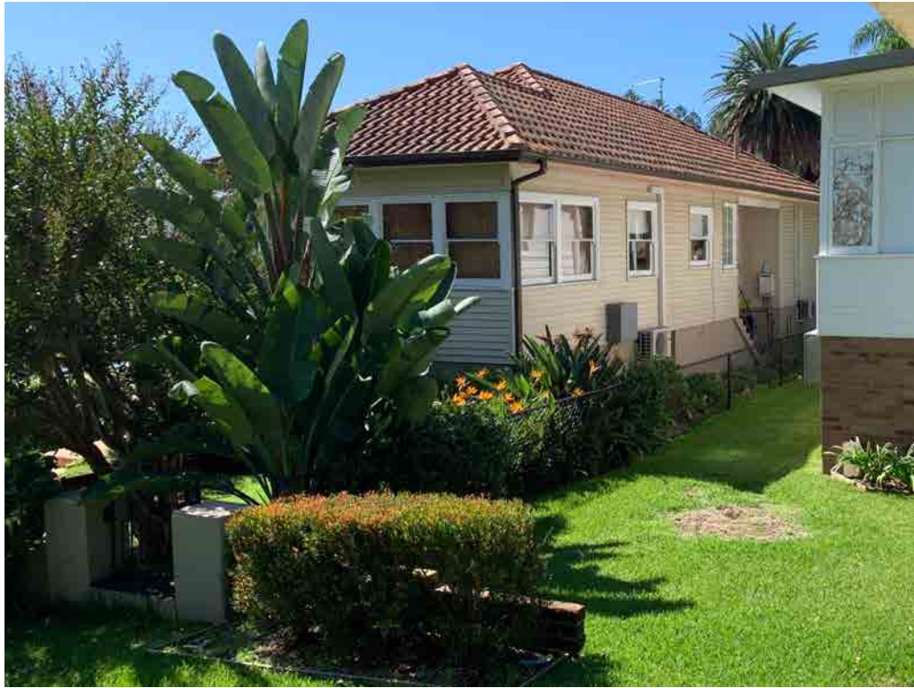
Interface with the northern boundary.
