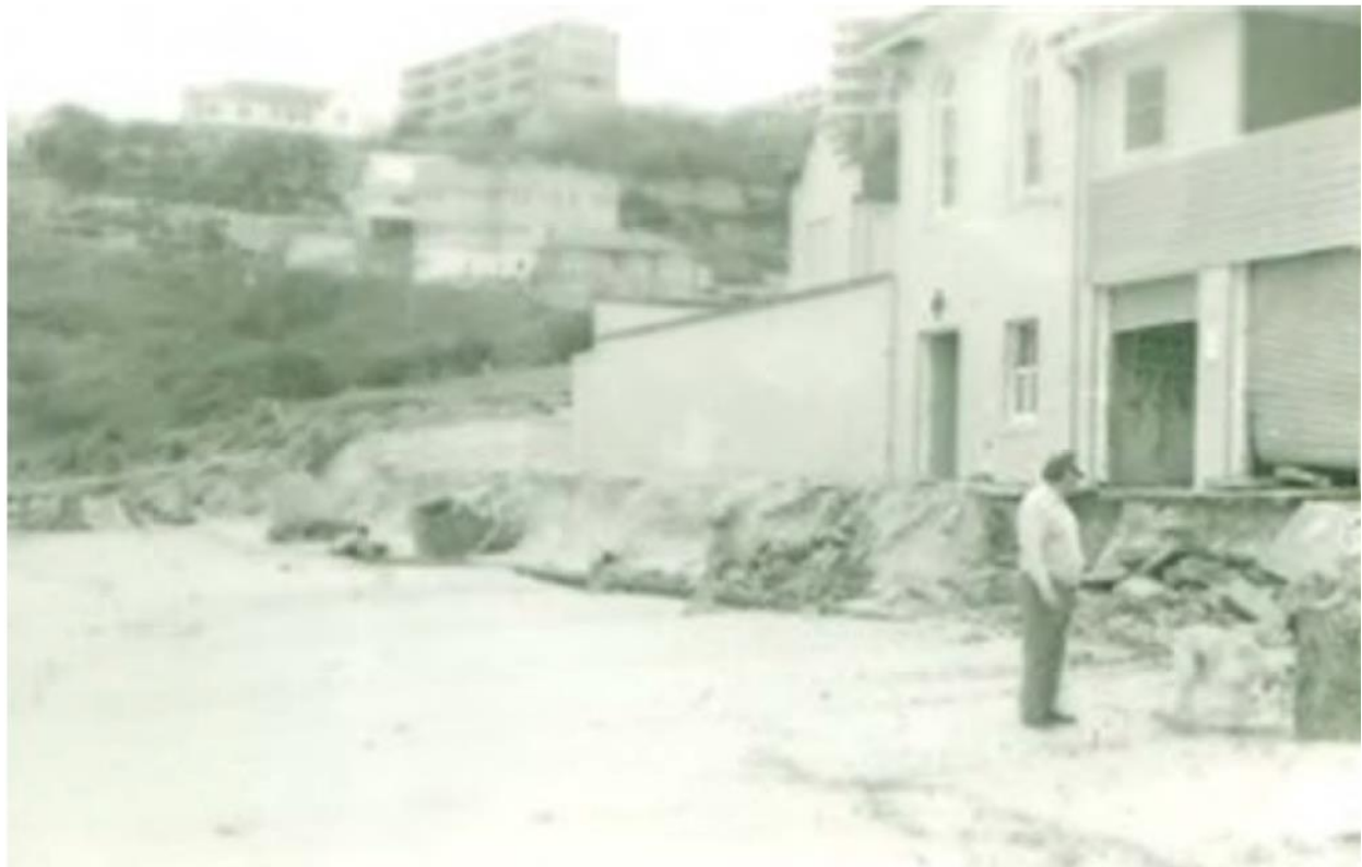
Figure 2-2 Erosion due to the 1974 storms and damage to the pavement and roller shutters (Source: UNSW Water Research Laboratory)
