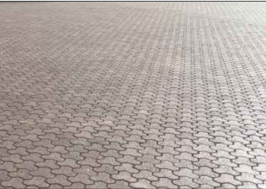
honed concrete 'Trihex' type pavers to new paved area on north side of building
