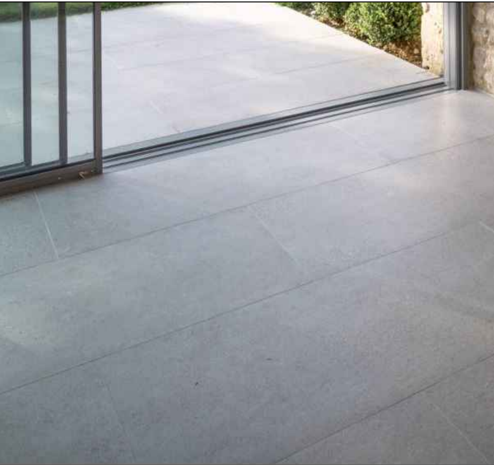
stacked sliding black satin powdercoated aluminum framed glass doors concept ie between new enclosed space on balcony and open balcony space
