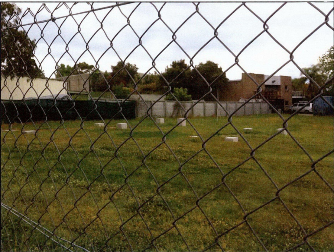
PHOTOGRAPH 2 - Photograph of Piers and Footings in North East corner of site
