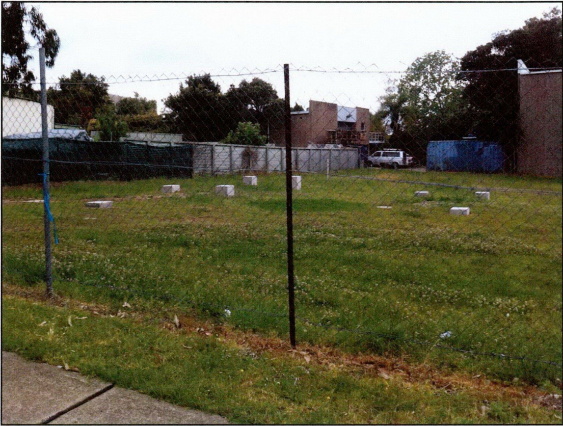
PHOTOGRAPH 1 - Photograph of Piers and Footings in North East corner of site
