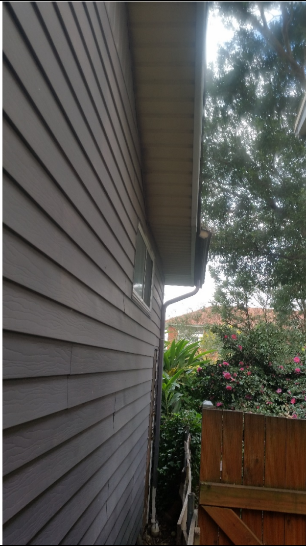
Figure: Gutter & drain over property boundary, eaves on or over boundary.
