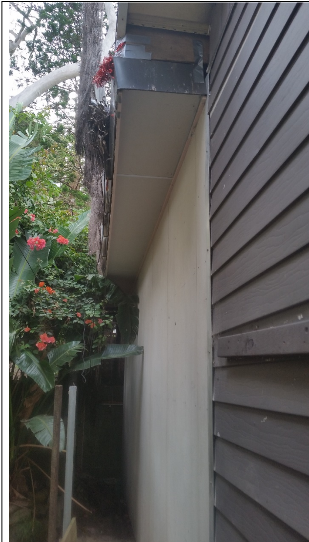
Figure: Roof not cut back as required.
