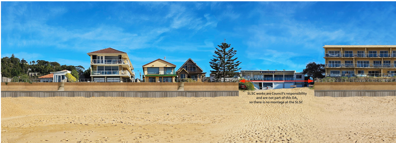
Image 2: Photomontage showing the works in a post storm state with sand scoured down to the cemented sand level (as low as it can go) and no vegetation.
