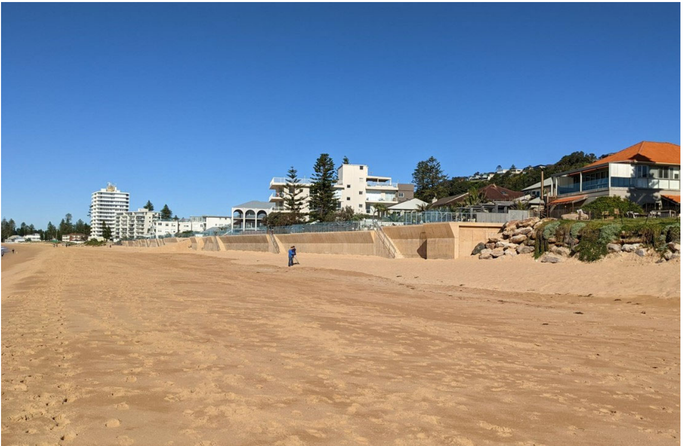
Image 4: An angled, morning, view of the two stretches of vertical wall already constructed between Stuart and Clarke Streets.
