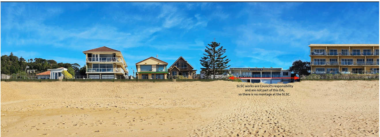
Image 1: Photomontage of the proposed works showing the median historical sand level with vegetation screening. The montage is made up of a series of images taken on 14 July 2023, approximately 40m from the eastern property boundaries. The beach was approximately 50m wide at the time the photos were taken.
