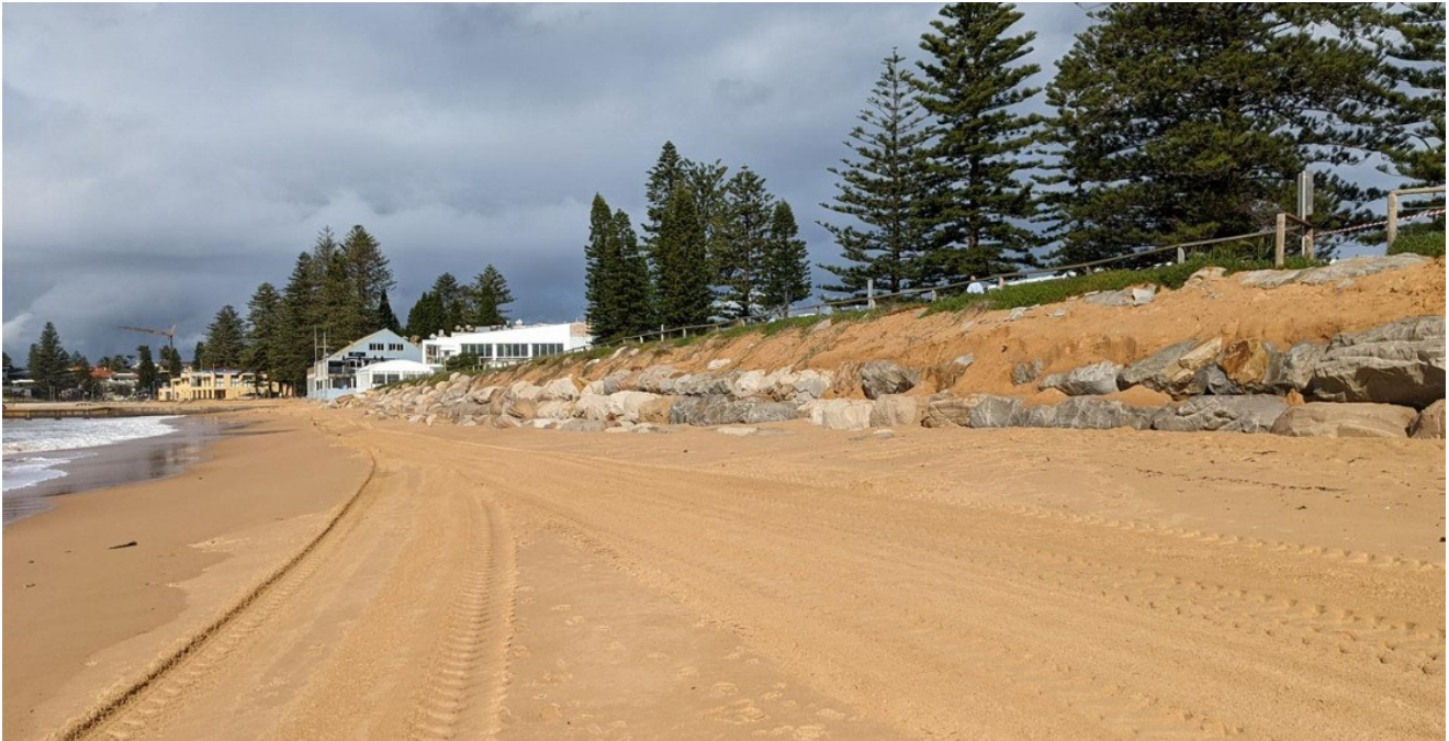
Image 6: View of the rock revetment wall protecting the Collaroy carpark.
