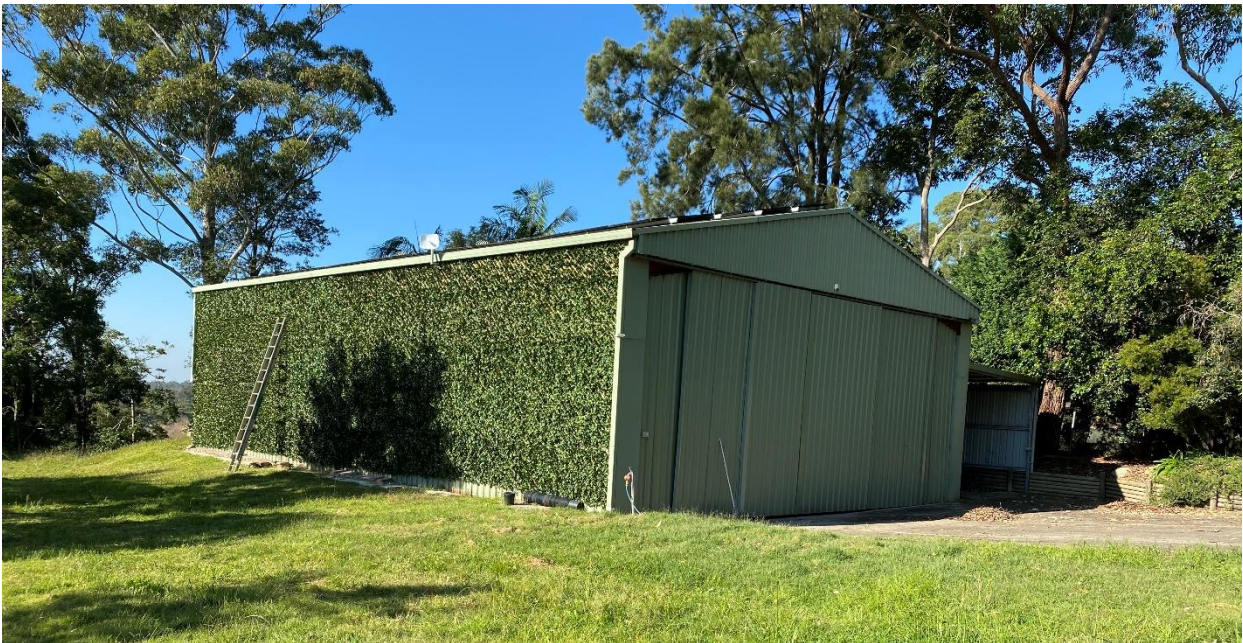
Figure 5. Image of the existing Barn / Workshop shed
