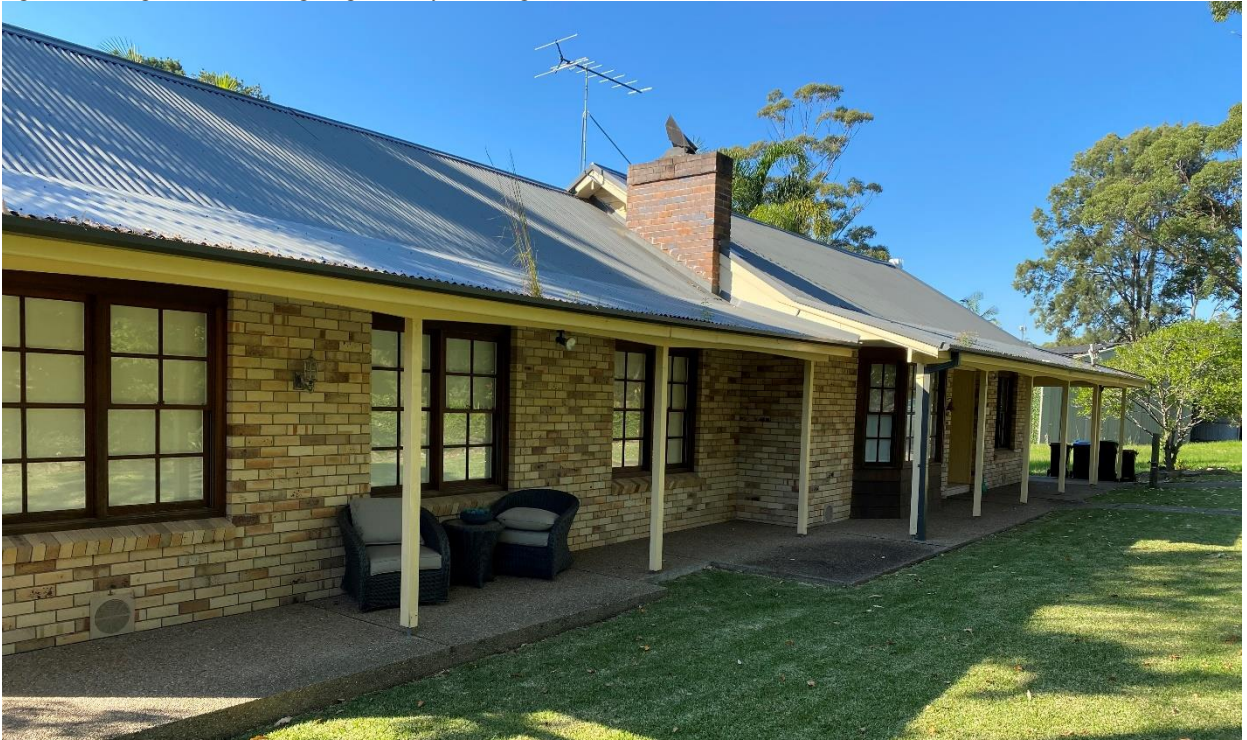
Figure 4. Image of the existing single storey dwelling
