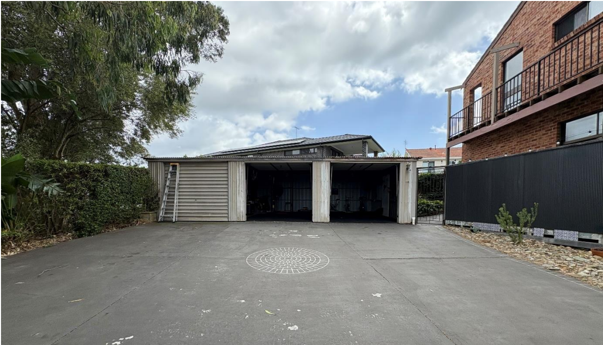
Figure 3: The existing garage, to be demolished, which will allow for secondary dwelling.
