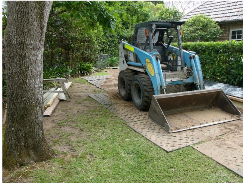
Figure 4 – Showing typical detail for truck mats.
